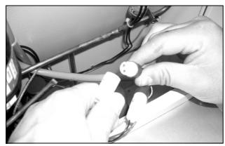
Fig. 67: Disconnect the fan connectors (3)
