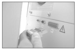
Fig. 53: Disconnect the mains plug
