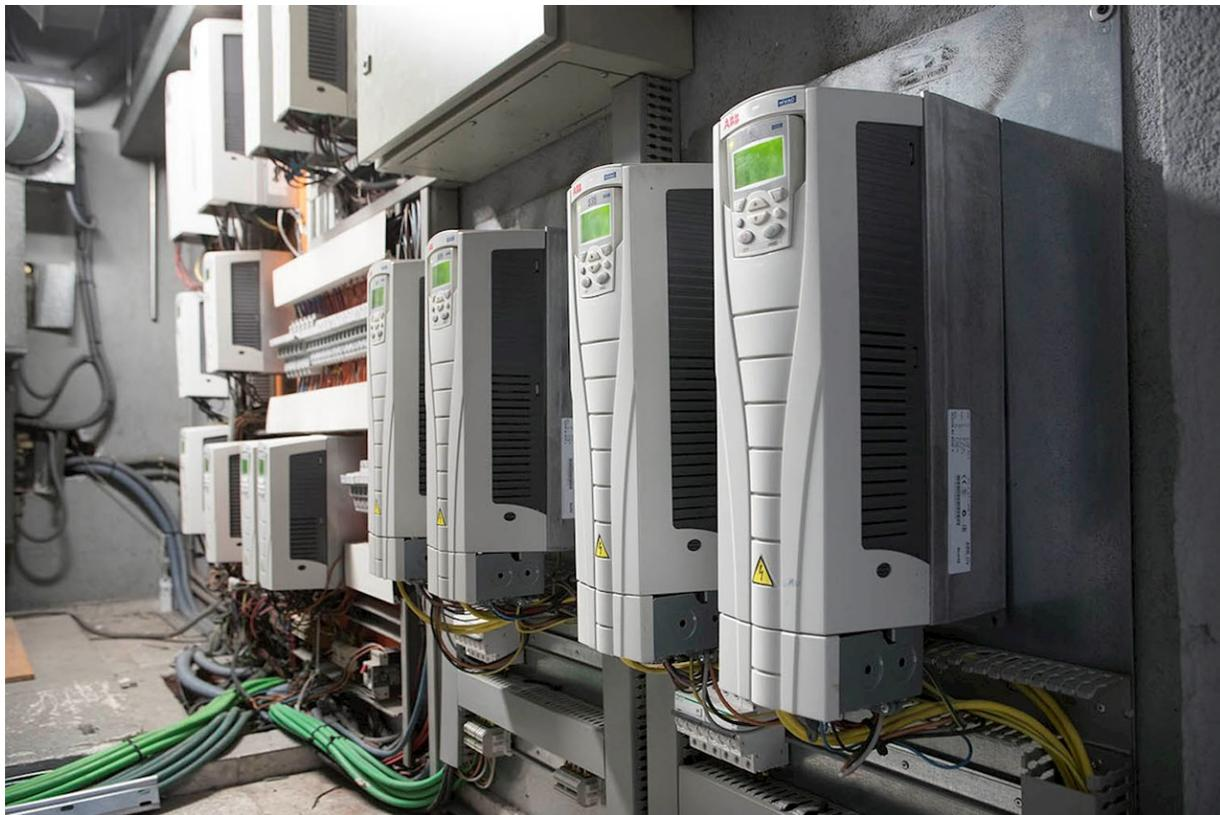
Based on these findings, the pumping systems were equipped with 13 ABB ACH550 variable speed drives (VSDs) and 16 electric motors with IE3 energy efficiency classification, and integrated into building management systems. This upgrade provides the overall system with greater stability and higher energy efficiency, as the motor speeds are now adjusted to match the precise demand at any given time.
